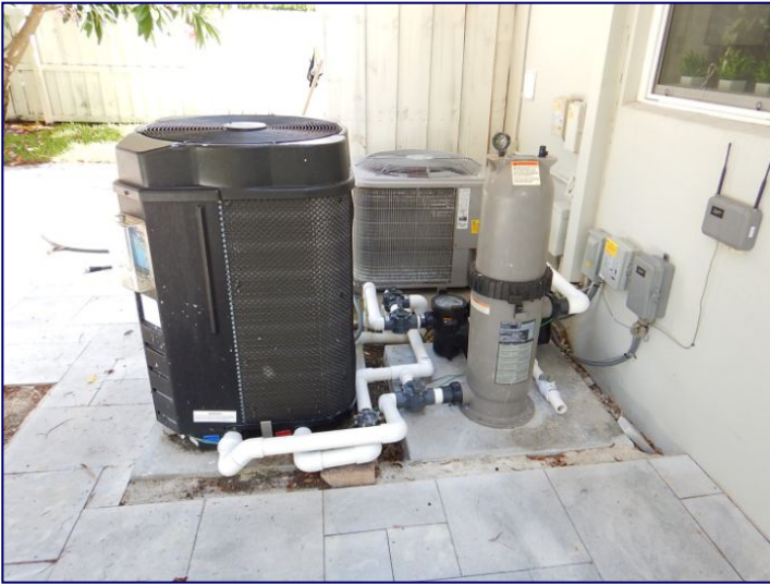
Pool motor/pump operated properly by the on/off switch and or timer at the time of inspection.
